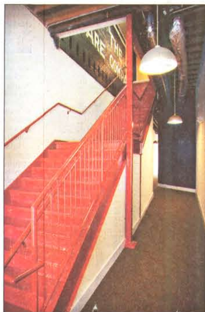
Part of a painted Standard Hardware sign is visible on the brick in this unit. The sign had to remain as part of the historic restoration.
